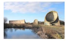
are large concrete structures, built in the late 1920s and early 1930s, designed as an early warning system for Britain to detect enemy aircraft. These worked by focusing the sound from the plane's engine so it could be heard before it was visible. There were three designs of mirrors, 20ft, 30ft and 200ft, and all three can be seen in Greatstone, located in the northeast side of the Dungeness Nature Reserve.
