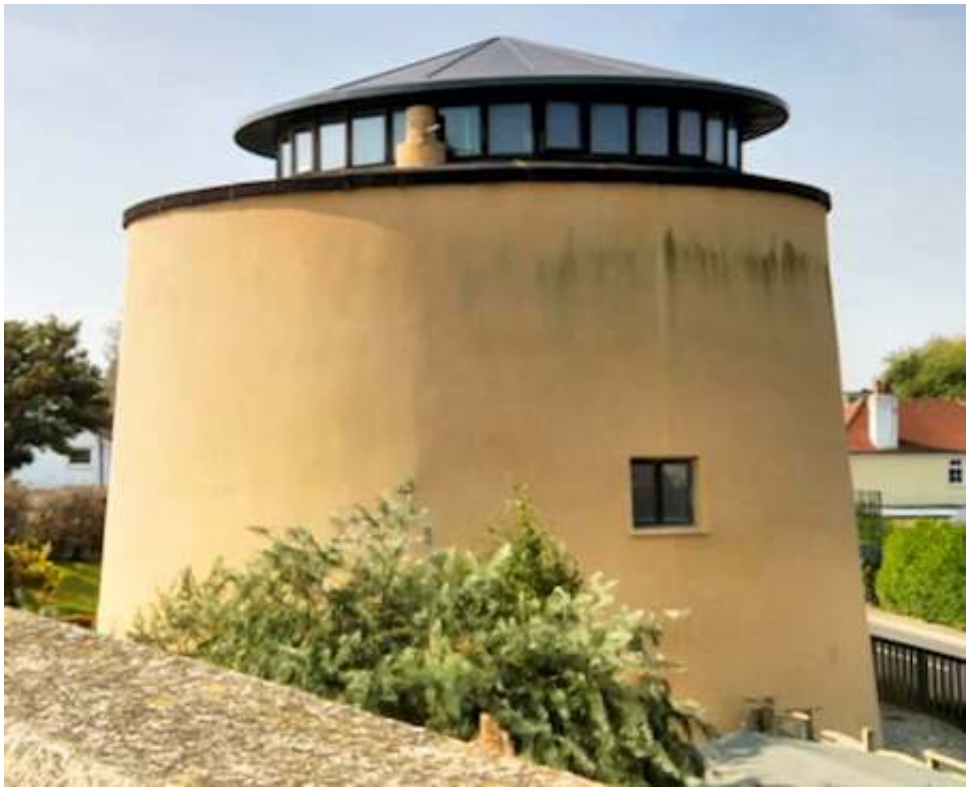
Martello Tower No. 23
