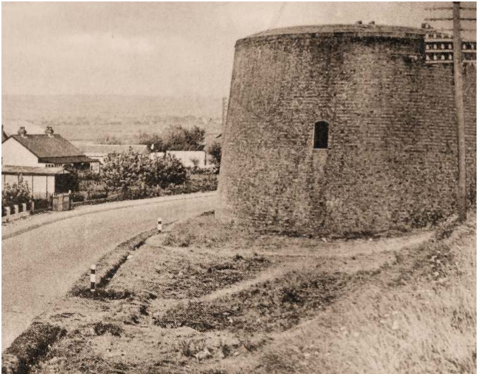
Martello Tower No.22 before it was demolished in 1956
