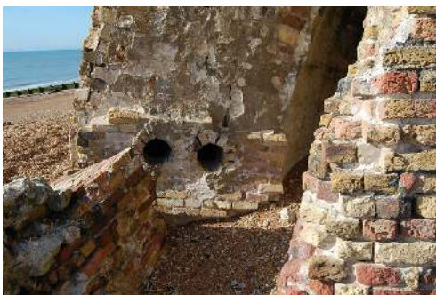
Showing the smoke/vent holes
